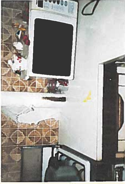
FIGURE 7-21 Fire damage on kitchen countertop at scene of fire. Note V pattern on paper towel roll and burn mark on microwave front window. Courtesy of Ross Brogan (ret.), NSW Fire Brigades, Greenacre, NSW, Australia.
